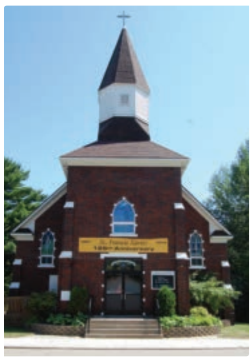
The exterior trim of St. Francis Xavier church was recently painted.
